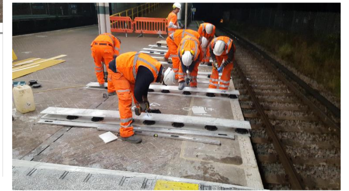
STAGE 3 FIXING PEDESTAL CAR PLATE
