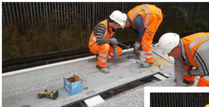
STAGE 5 FIXING COVER AND EDGE TACTILE
