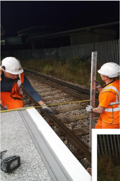
STAGE 4: SETTING COVER EDGE TO GAUGE
